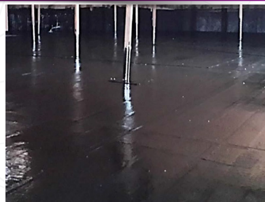
▲ Petroleum storage tank after reinforcement by laminated composites
